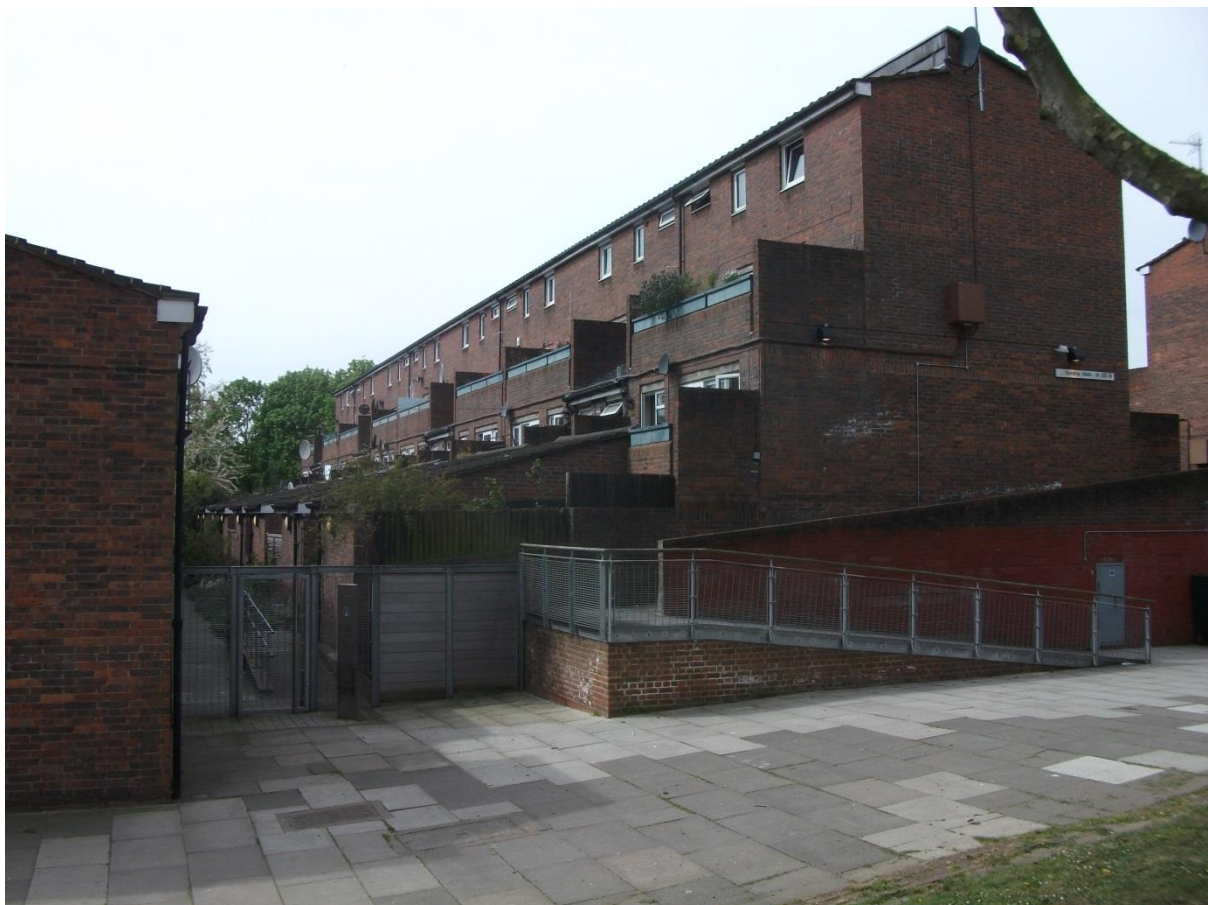
Figure 1 Balconies above bedroom and hallway and pitched roof above the living room to the ground floor flat entrance. Elevation of a typical four storey block with individual garages behind.
