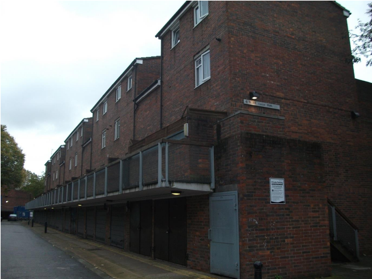
Figure 2 Typical four storey block- with individual garages at ground floor level. These back directly onto the ground floor one bedroom flat units.
